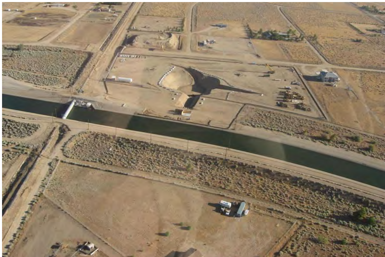
Neenach Temporary Pumping Station, construction site, looking northerly, taken September 16, 2010, by Aqueduct Aerial Patrol.
